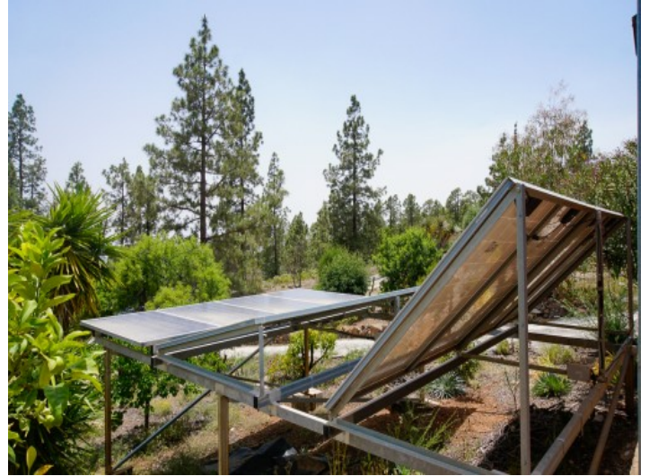
Large solar panels
